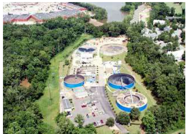
Daphne Utilities' Water Reclamation Facility had space limitations for new equipment
