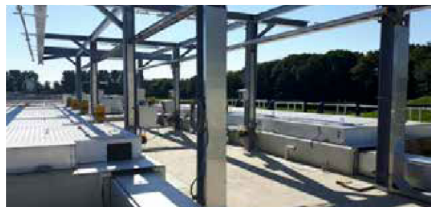
Eight SFK600 Salsnes Filters installed into channels
